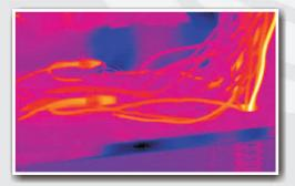
A ground wire short is detected with an Infrared camera. The ground wire is carrying 20 amps.
